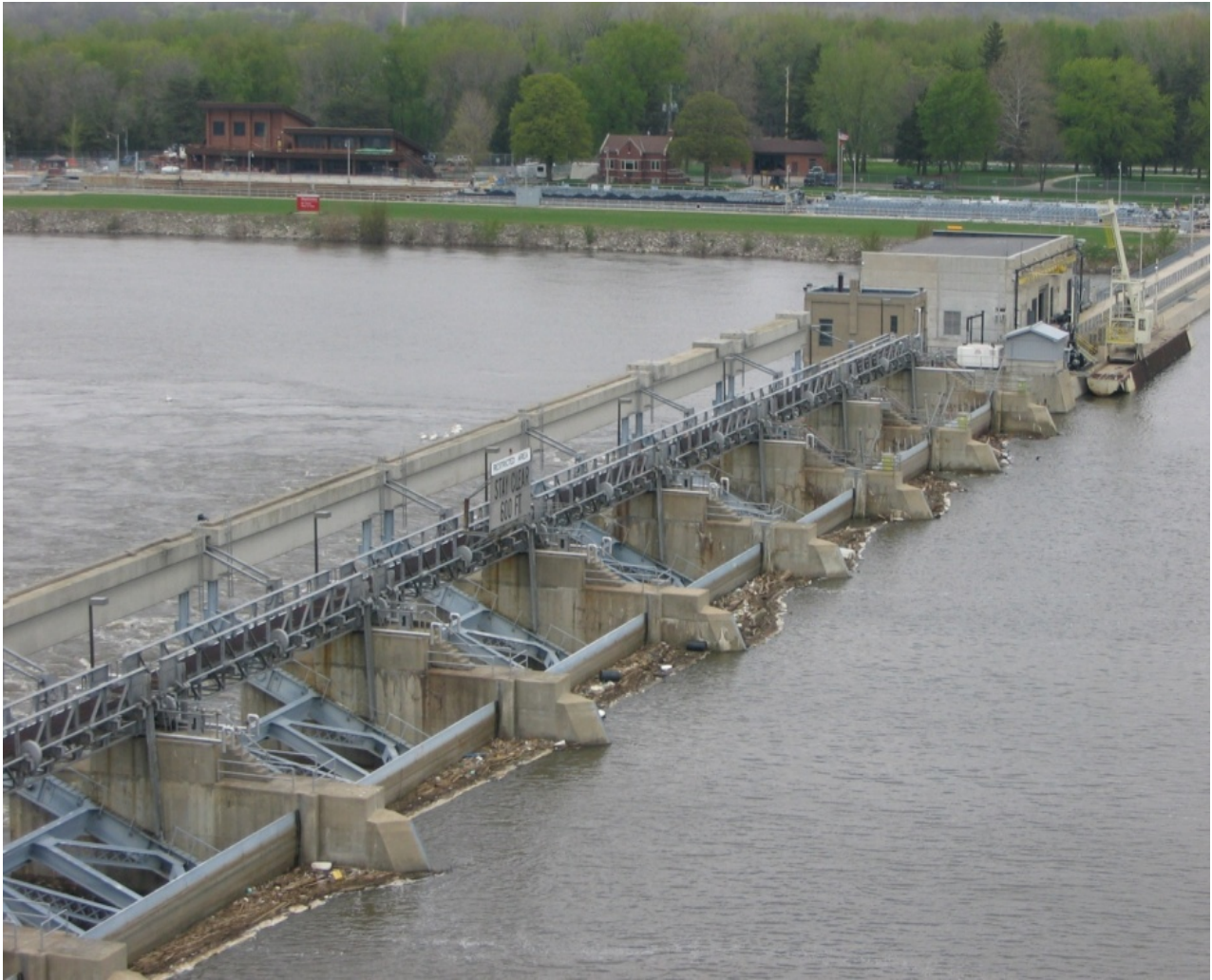
Fig. 3 Starved Rock Lock and dam on the Illinois River waterway.
