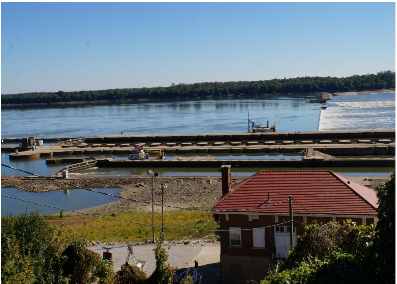
Fig. 7 Lock and dam number 53 on the Ohio River near Olmsted, Illinois.
